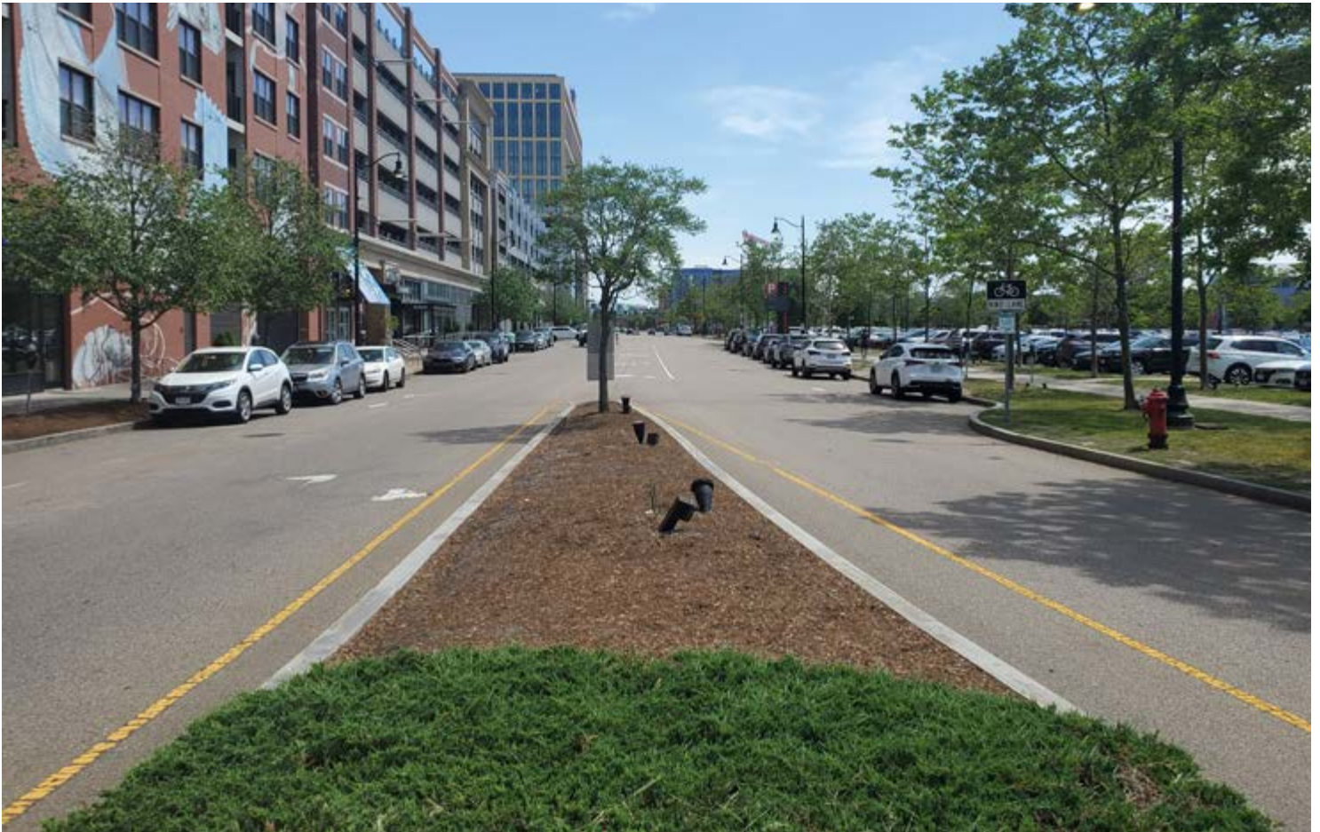
Looking south from Grand Union Blvd. and Greater River Rd. illustrates this parking problem. On the left are two multi-story car parks, and on the right is a 5.6 acre parking lot. (Source: Peter Ciurczak)
