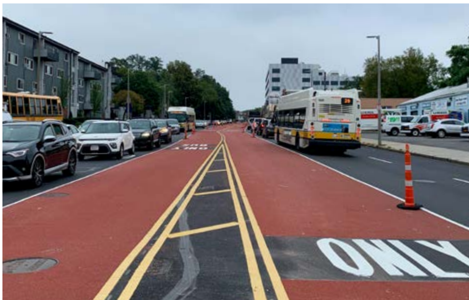
Center running dedicated bus lane on Columbus Ave. (Source: Trevor Mattos)
