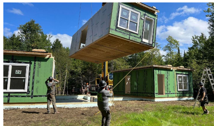
ADU under construction.
