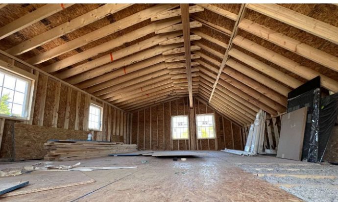
ADU under construction.
